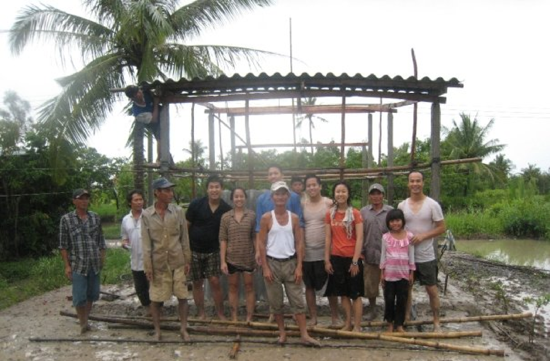
Build house for the poor in Cà Mau
